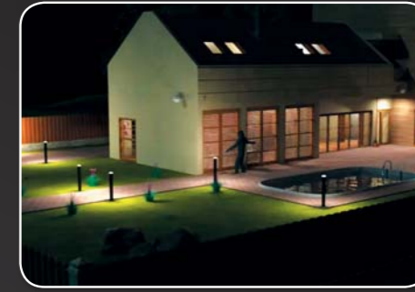
Alarm lighting activated when the building is disturbed.
